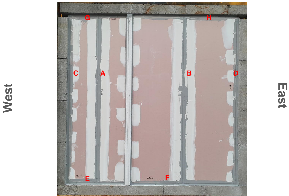
Figure 24 Unexposed face of the specimen before the start of the test
